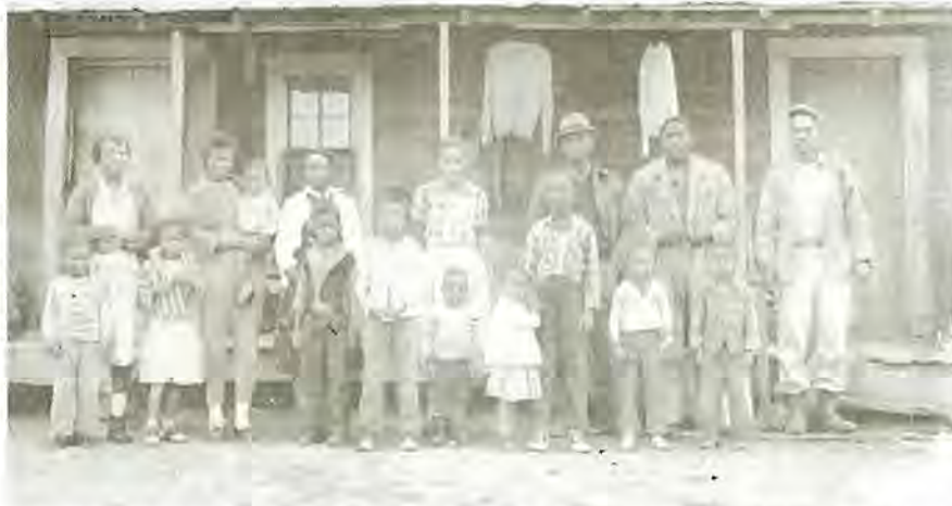
This is the dilapidated housing provided for day workers and others in Fayette County and this is "home sweet home" for all of those in the above photograph.
